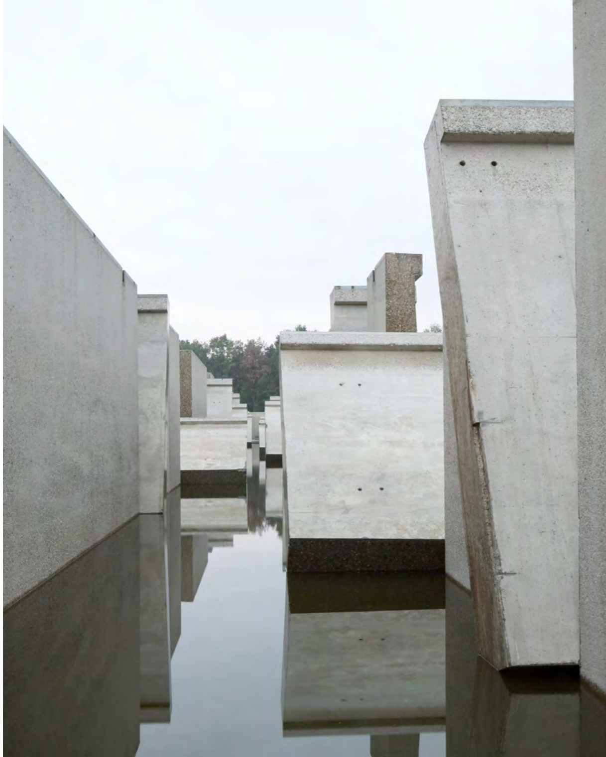
Deltawerk // Concrete has been sand blasted to open up the toplayer as a habitat for mosses, lichen and ferns
