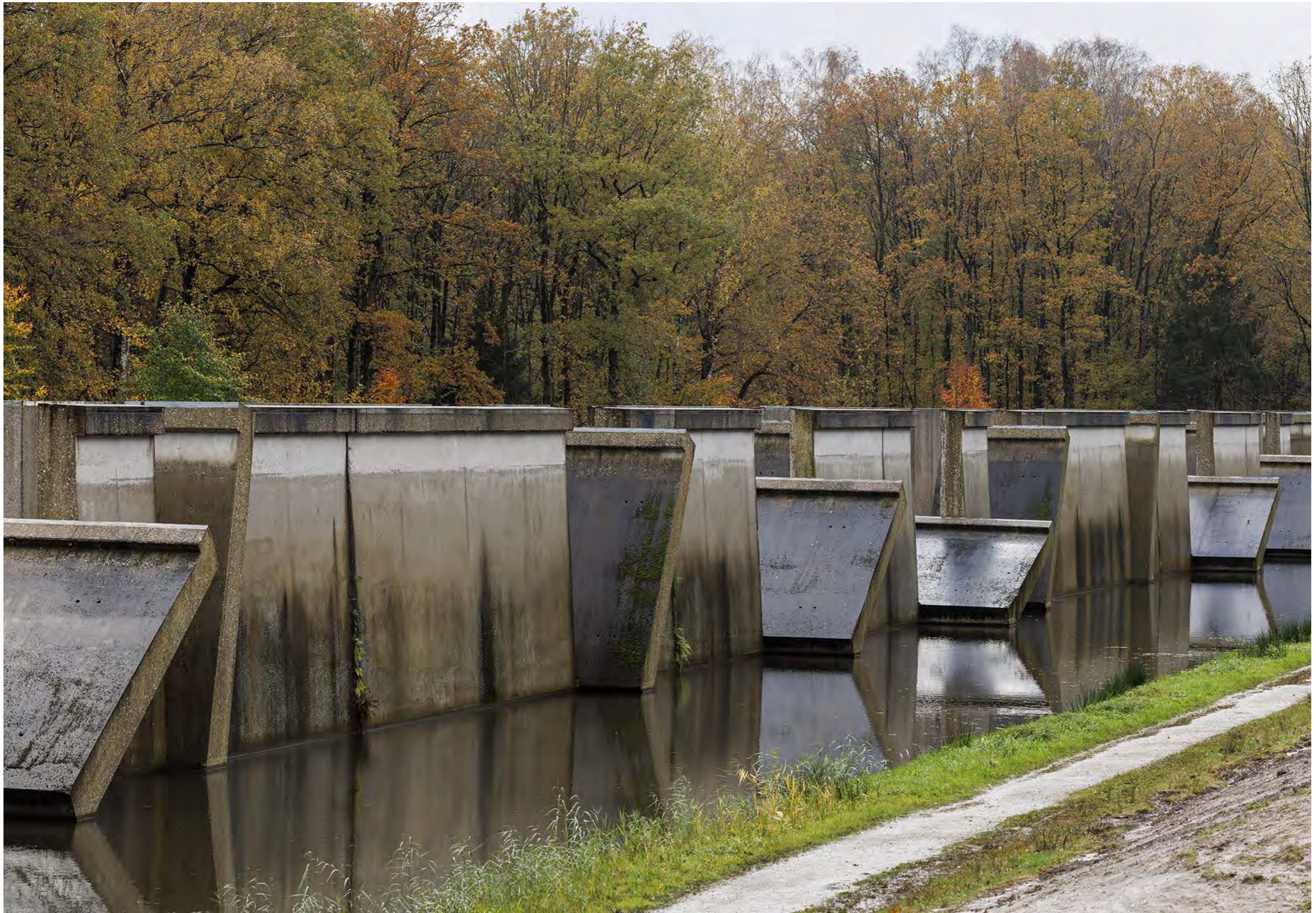
2023 Mosses, ferns and lichen start to grow at the sandblasted concrete skin
